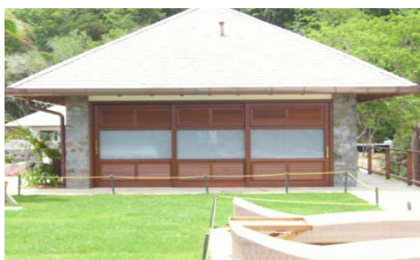
Media Room and Pool Bar- during the construction process, and finished.
